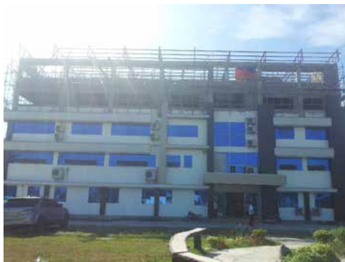
Picture 8. Frontage of the five-story structure of the MGWPAC (photo taken during research site visit on 8 December 2015).
